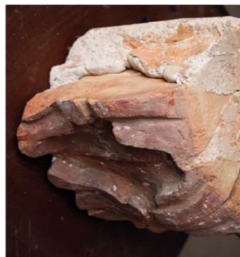
Figure 9: A part of a bricked head column.
