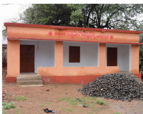
Figure 4: The clinic as in Figure 3a was disbandeld and this new structure was brought up. Alas! After completion, it was announced that IRCS clinic is no more. This tenement was allotted to the engineering division.
