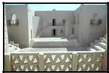
Figure 4: Patterns in the parapet wall (Iskander).
