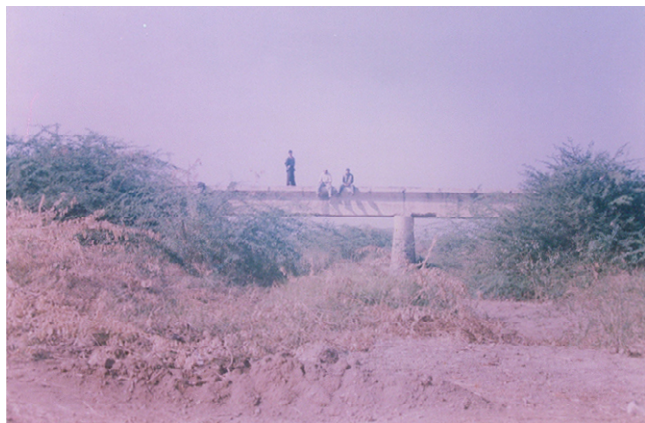
Figure 13: Aqueduct over Mota Thordi Nadi for abandoned canal.
