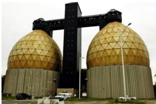
Figure 4: Back River Wastewater Treatment Plant.
