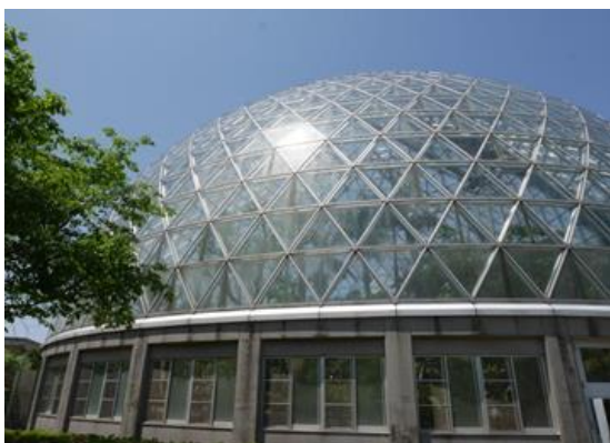
Figure 5: Niigata Prefectural Botanical Garden.
