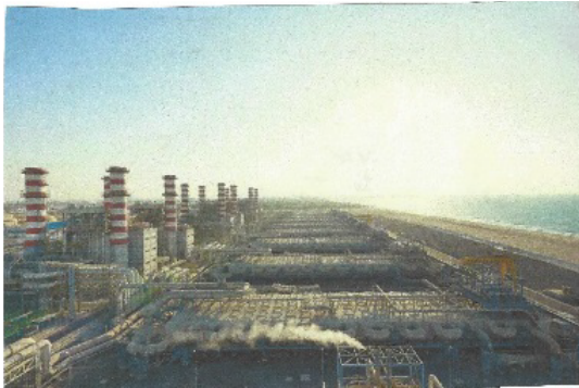
Figure 11: Fujairah's water desalting town.
