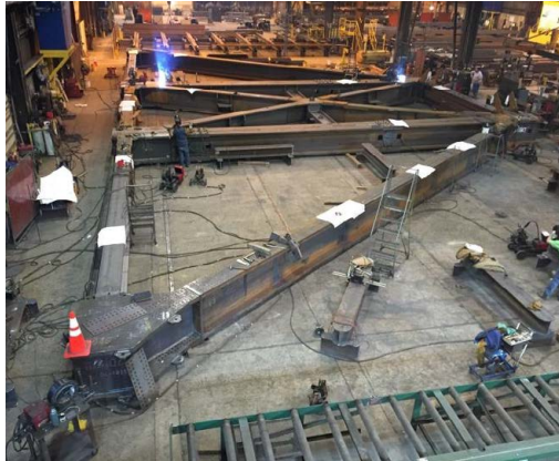
Figure 23: Pre-Assemble in fabrication shop.
