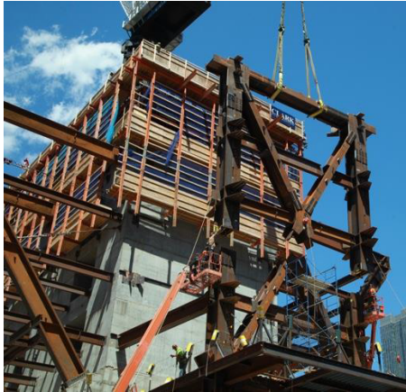
Figure 18: Heavy Steel assembled truss erection at high level.
