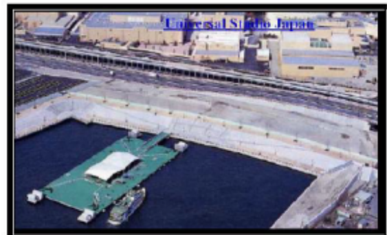
Figure 4: Emergency rescue base in Osaka bay.
