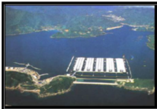
Figure 2: Kamigoto floating oil storage base, Nagasaki prefecture, Japan.
