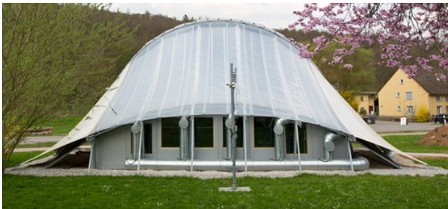
Figure 2: The polar bear pavilion, inspired by the solar thermal functions of the polar bear's fur.
