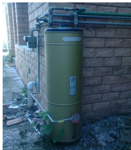
Figure 2: Gas geyser connected to the output of the solar geyser (hybrid gas geyser).
