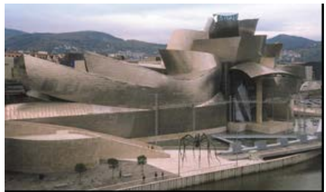
Figure 7: in this building the structure follows form being hidden beneath form layers.
