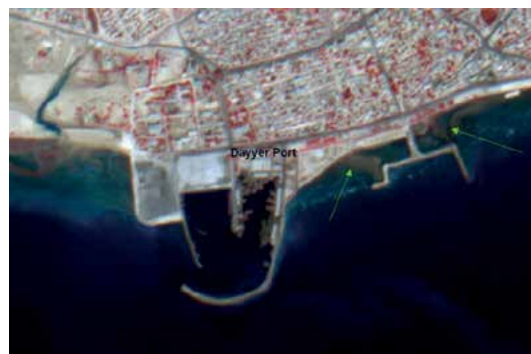
Figure 10: Deposition of sand in Dayyer Port.
