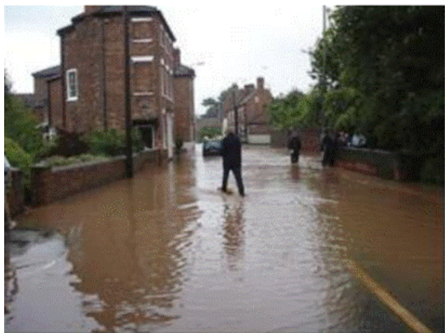
Figure 3: Flooding in Coventry [8].
