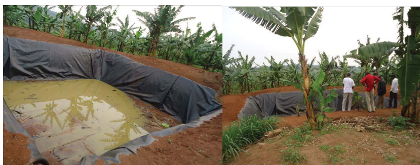
Figure 18: Rain water collection method using polythene sheet on the ground.
